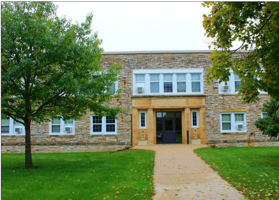
Pollard Hall is one of many state academy buildings eyed for improvements.
